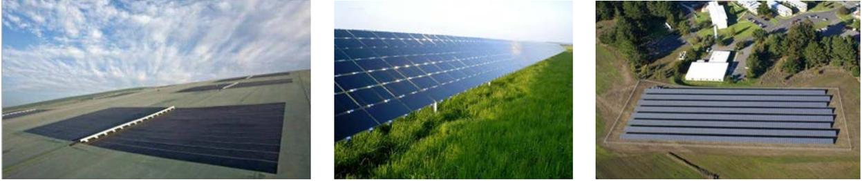
**Figure 5. Thin-film solar panels installed on (left) solar energy cover and (middle/right) fixed-tilt mounting system. Photos by (left) Republic Services Inc., NREL 23817, (middle) Beck Energy, NREL 14726, and (right) U.S. Coast Guard Petaluma Site, NREL 17395**
